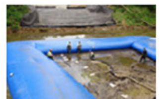
Cofferdam Dredging 围堰疏浚
