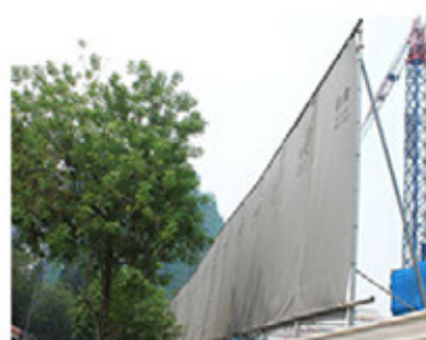
Railway sides 铁路两侧
